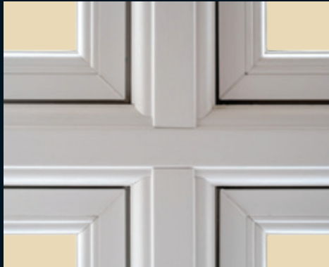
Arrissed joints mimicking traditional timber joinery
