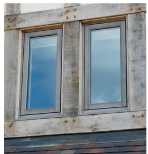
New complementing the old Dummy or functional stays upgrade
