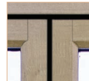
Mechanical joint upgrade
