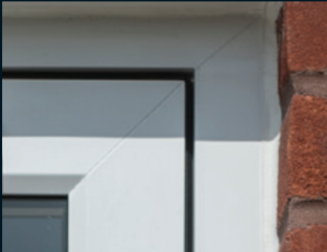
Standard - Corners welded (sash and outerframe)
