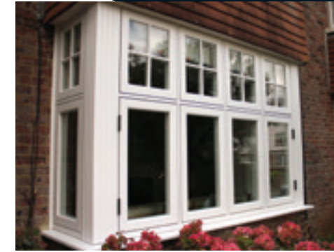
Flush external finishes with equal sightline
