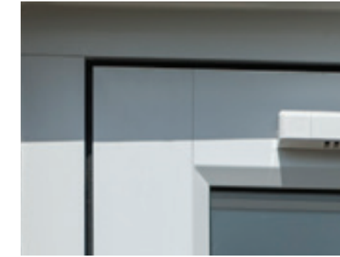
Timberweld jointed sash and outer frame
