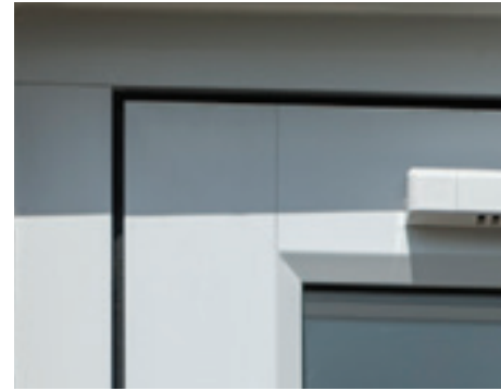
Timberweld jointed sash and outer frame
