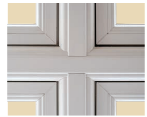
Arriased joints mimicking traditional timber joinery
