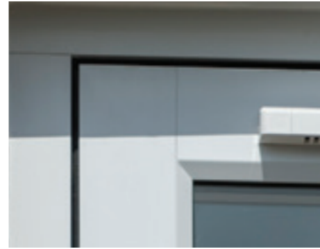
Timberweld jointed sash and outer frame
